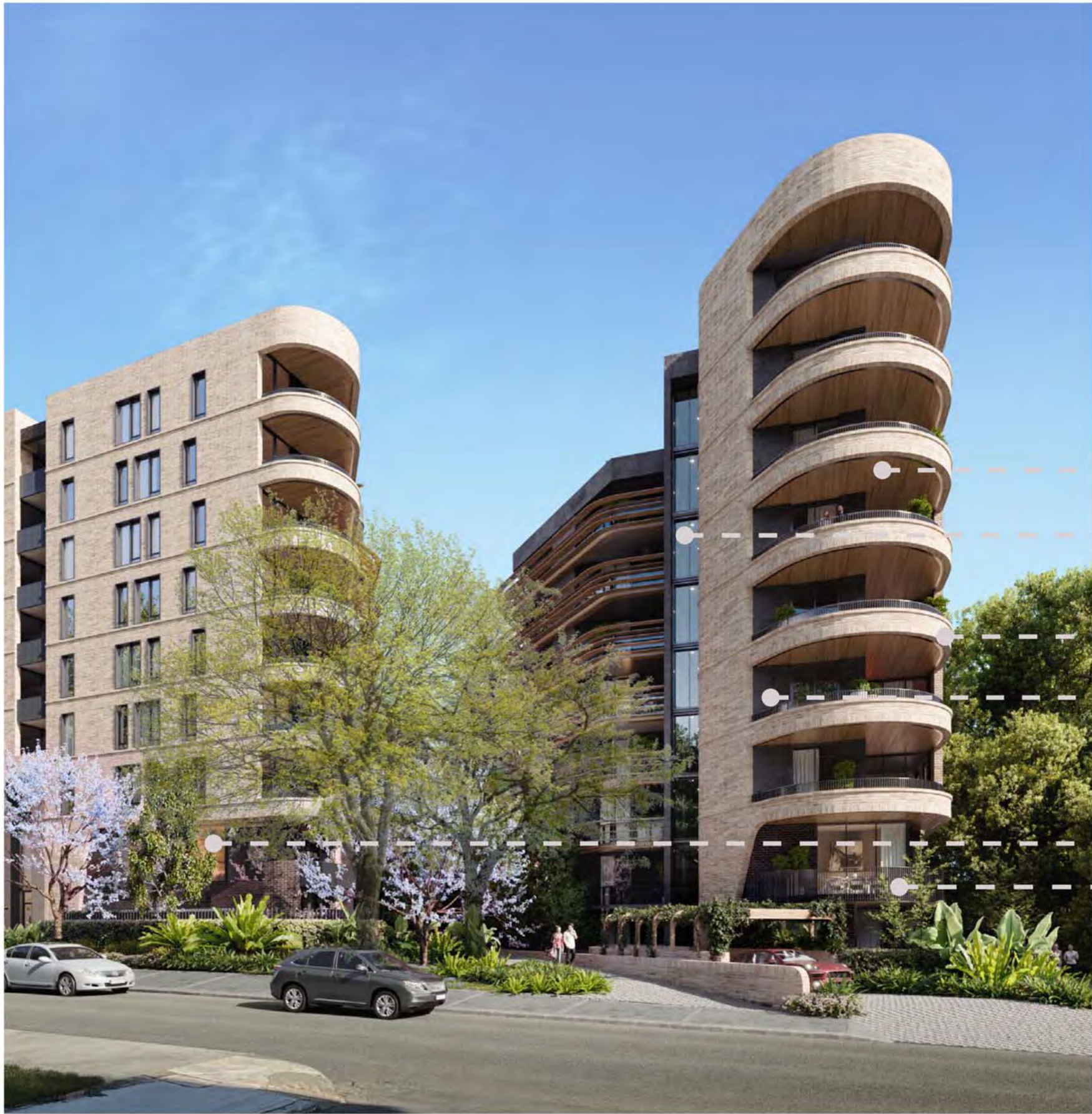
View from Northeast Corner
